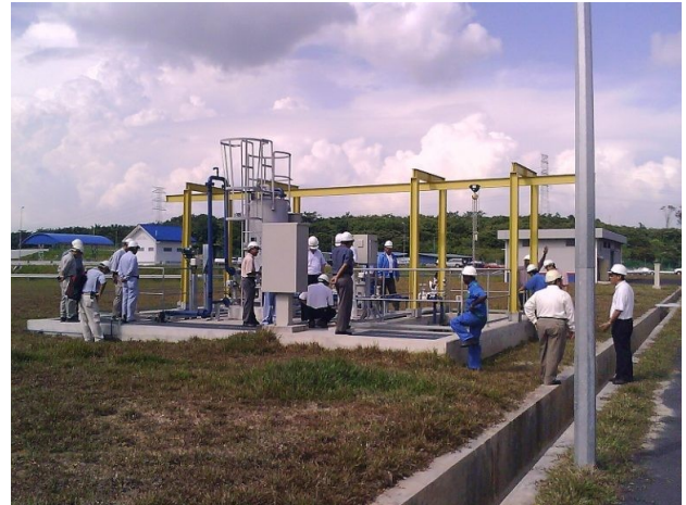
Sungai Udang Sewage Treatment Plant, Melaka, Malaysia
