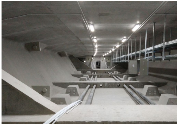
Inside view of the bridge.
